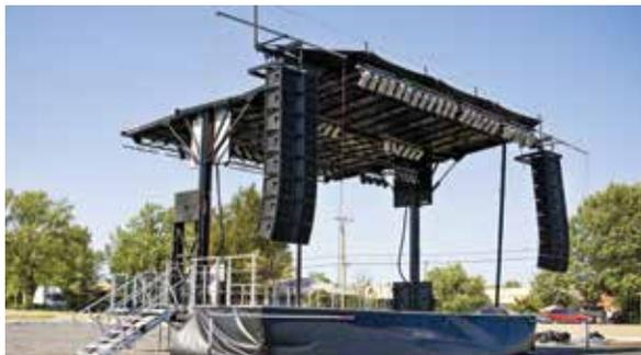
4 Roof & equipment fully raised. Install stairs, guardrails and add accessories.
